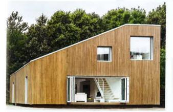
WFH house (above) constructed from repurposed shipping containers for the structure that can be combined to create a variety of open-plan living options. The carbon-neutral dwellings are easily demountable, include low-energy consumption materials and features, and require just a short construction period. Online tools allow customisation of the layout and the facade, on which sustainable materials can be used such as bamboo cladding, arcgency.com; worldflexhome.com
